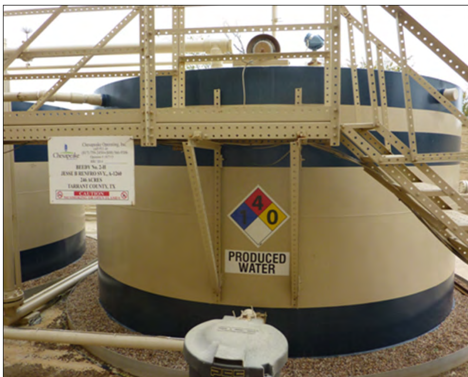
Figure 12: Storage Tank for Produced Water in the Barnett Shale
