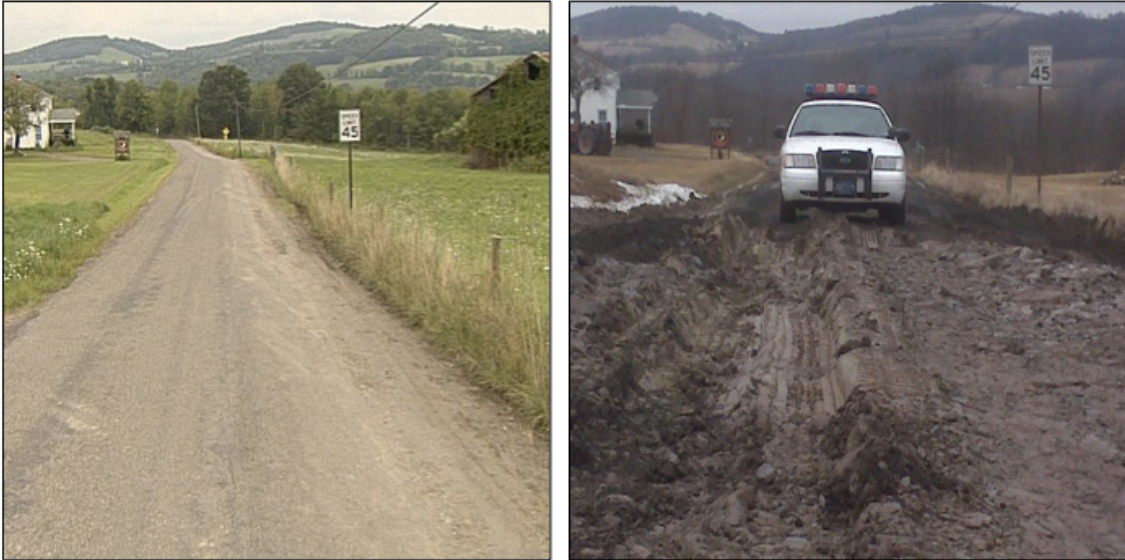
Figure 5: Before and after photos of SR 3020 in Bradford County, PA, due to heavy truck traffic during the dynamic spring thaw. Source: PA DOT.
