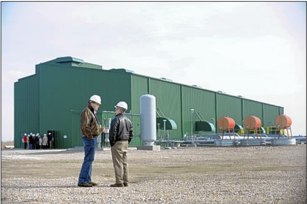
Gas Compressor Station
