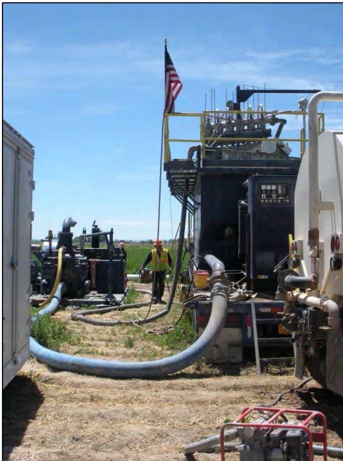
Figure C12. Photograph of flow of mud and cuttings to shakers at MW02.
