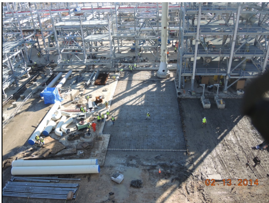
Train 2 131M01 (heavies removal unit paving) (13-Feb-2014)
