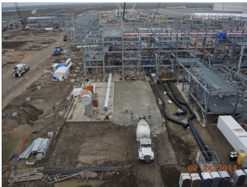
Train 1 131G02 (inlet gas-seal slab for paving) (24-Feb-2014)
