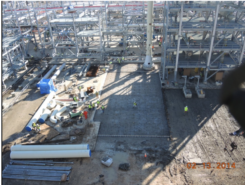
Train 2 131M01 (heavies removal unit paving) (13-Feb-2014)
