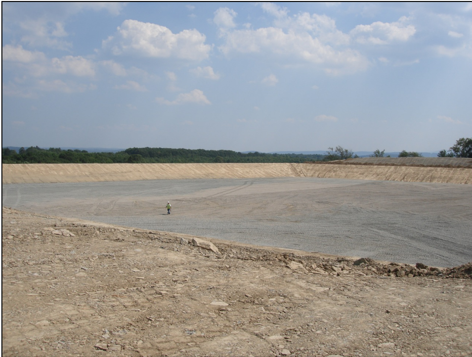
Well Pad Preparation (photo Carol Chock)
