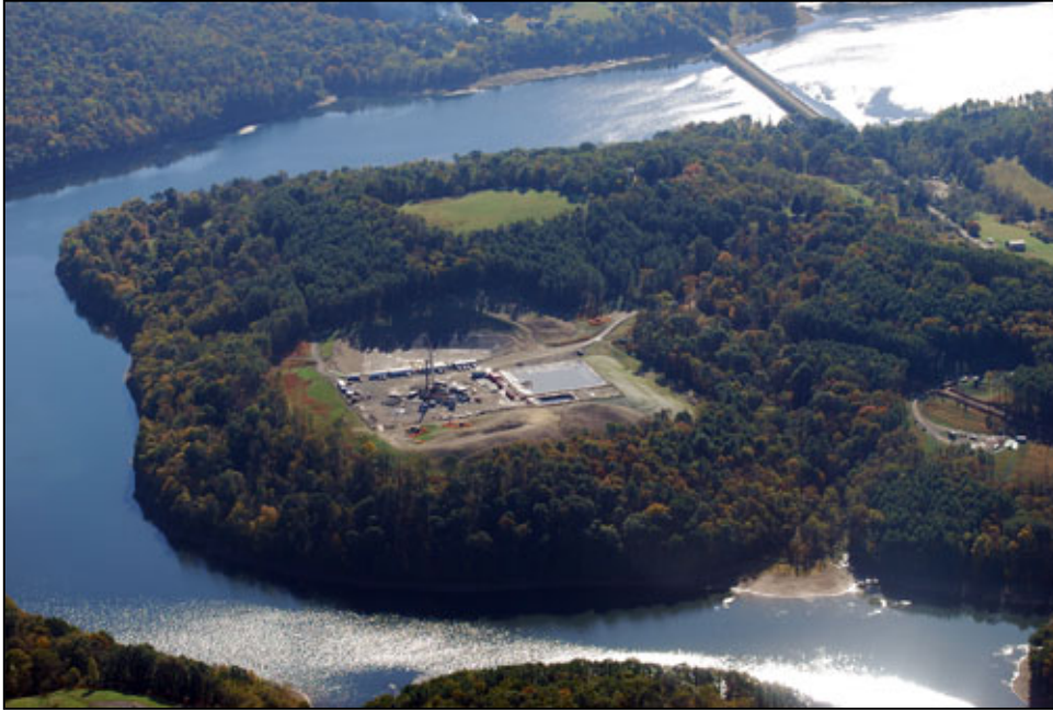
Well pad from scenic overview in PA
