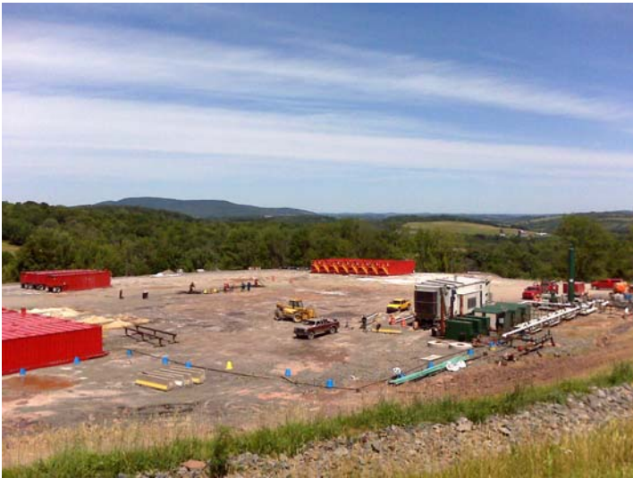
Photo 5.26 Fortuna multi-well pad after hydraulic fracturing of three wells and removal of most hydraulic fracturing equipment. Production equipment for wells on right side of photo. Source: Fortuna Energy, July, 2009.
