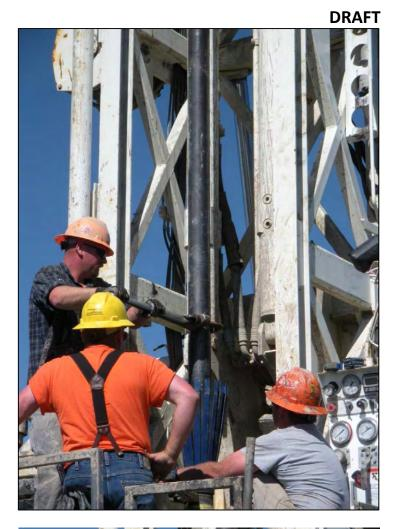
**Figure C21.** Photograph of securing sand basket and casing above screen.
