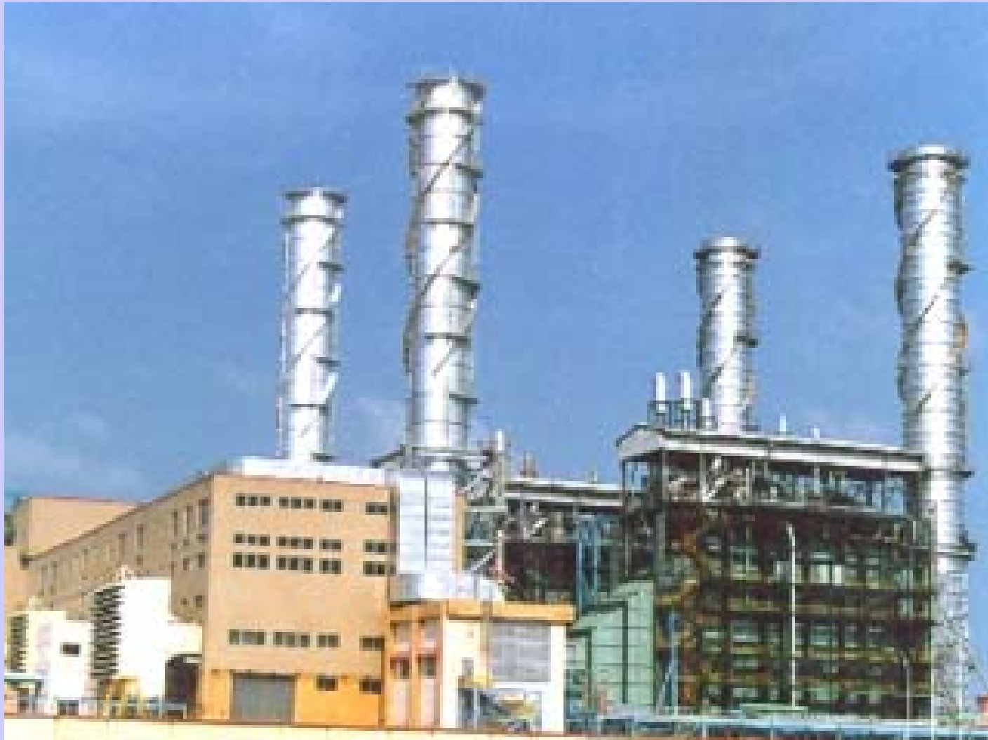
Combined Cycle Plant of BHEL
