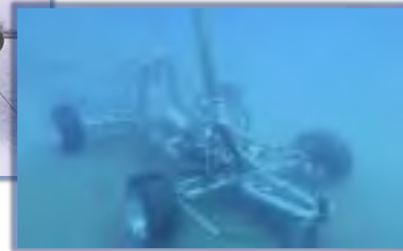
Cable burying machine (water-jet tool)
