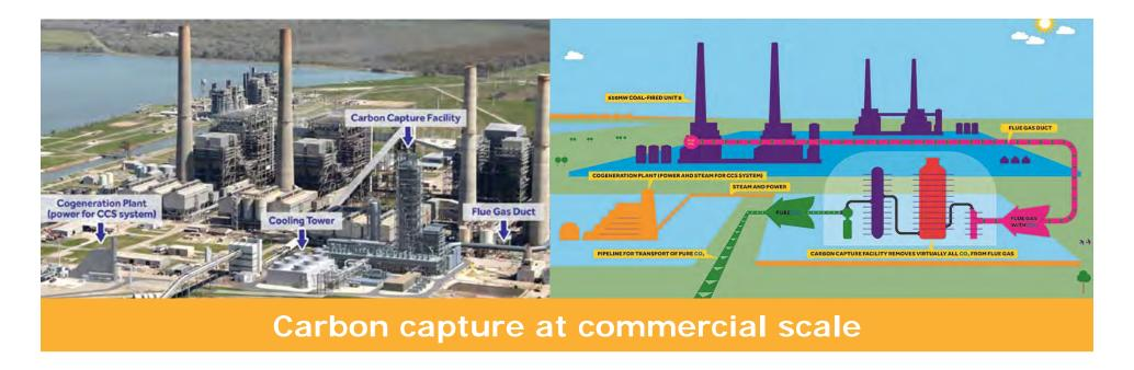
We are building the world's largest post-combustion carbon capture-enhanced oil recovery project
