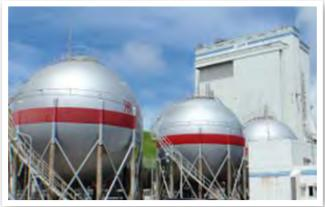
Largest liquefied hydrogen tanks in Japan (Tanegashima Rocket Base)
