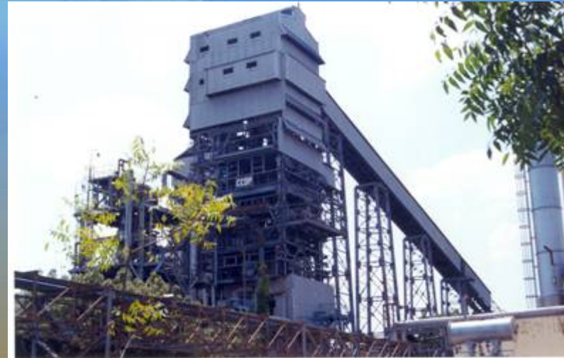
IGCC demonstration unit at Truchy
