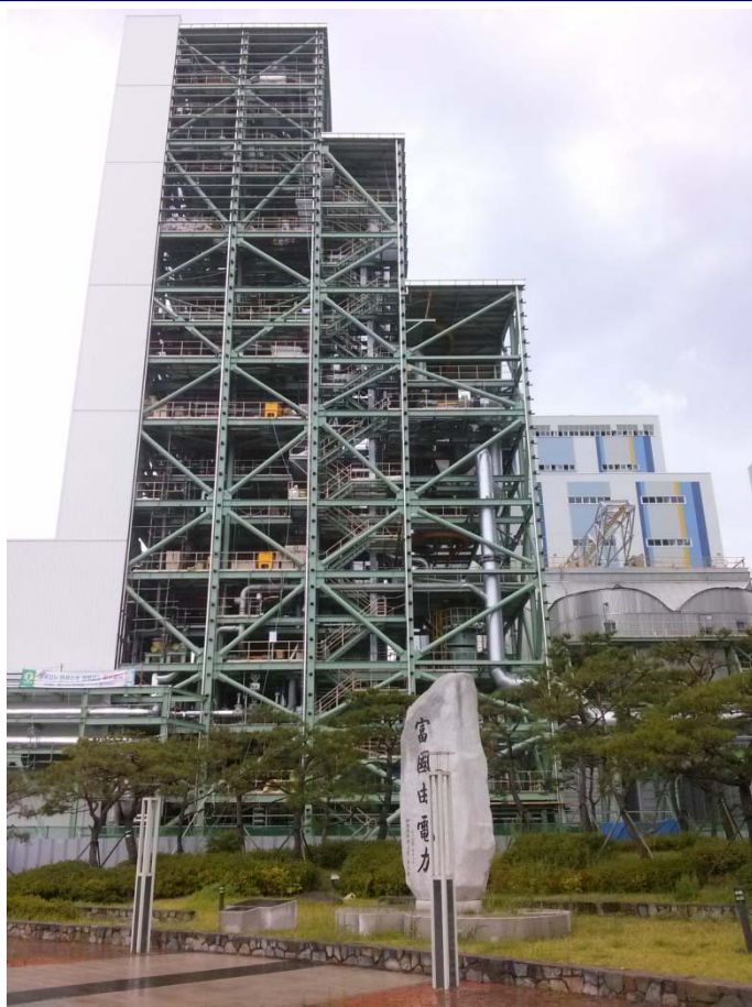
10 MW Pilot Plant at KOSPO's Hadong coal-fired power plant, Unit # 8
