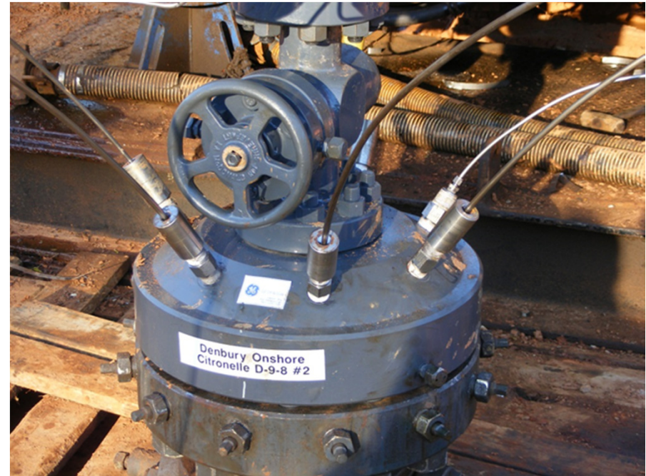
D9-8 wellhead as completed with control lines penetrating through port collars and collar sleeves.
