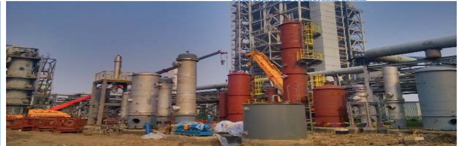
10000 CO 2 /year precombustion facility Palladium membrane H 2 /CO 2 separation system
