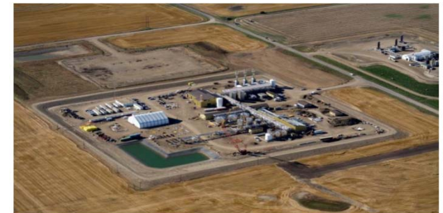
Aerial view of Pikes Peak South heavy oil thermal facility Courtesy: Husky Energy
