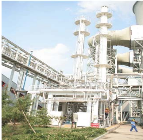
3000 tons CO 2 /year post-combustion Capture In Beijing
