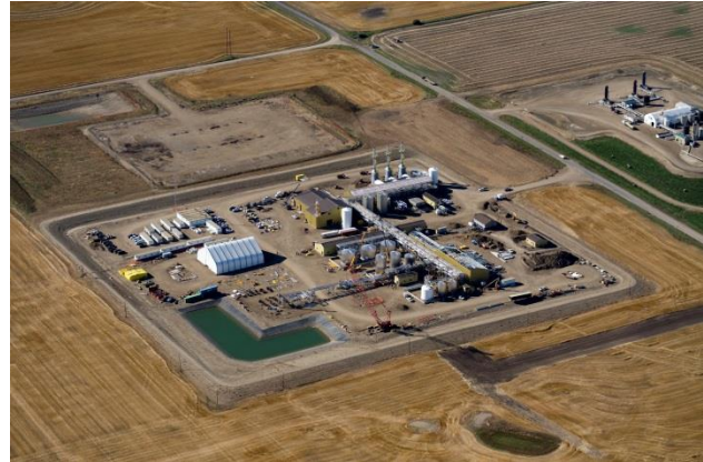
Aerial view of Pikes Peak South heavy oil thermal facility
