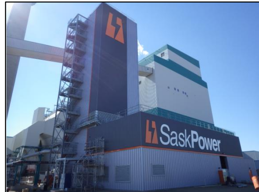
Shand Carbon Capture Test Facility (CCTF) - Estevan, Saskatchewan, Sept 2014 Photo Credit: SaskPower
