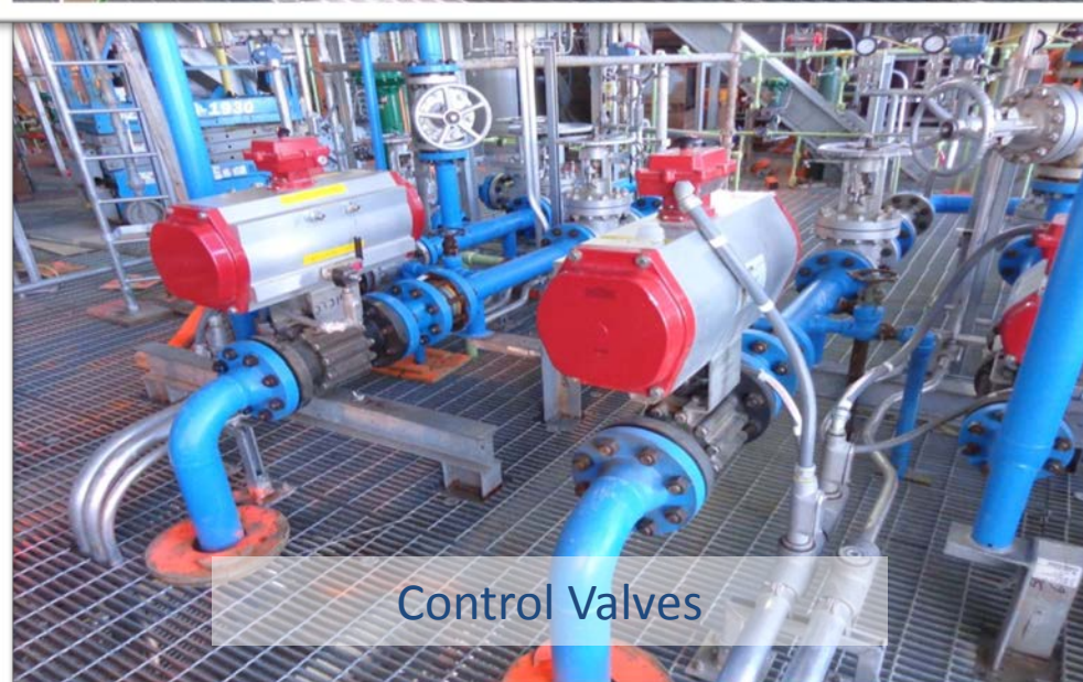
Steam Piping from Syngas Coolers
