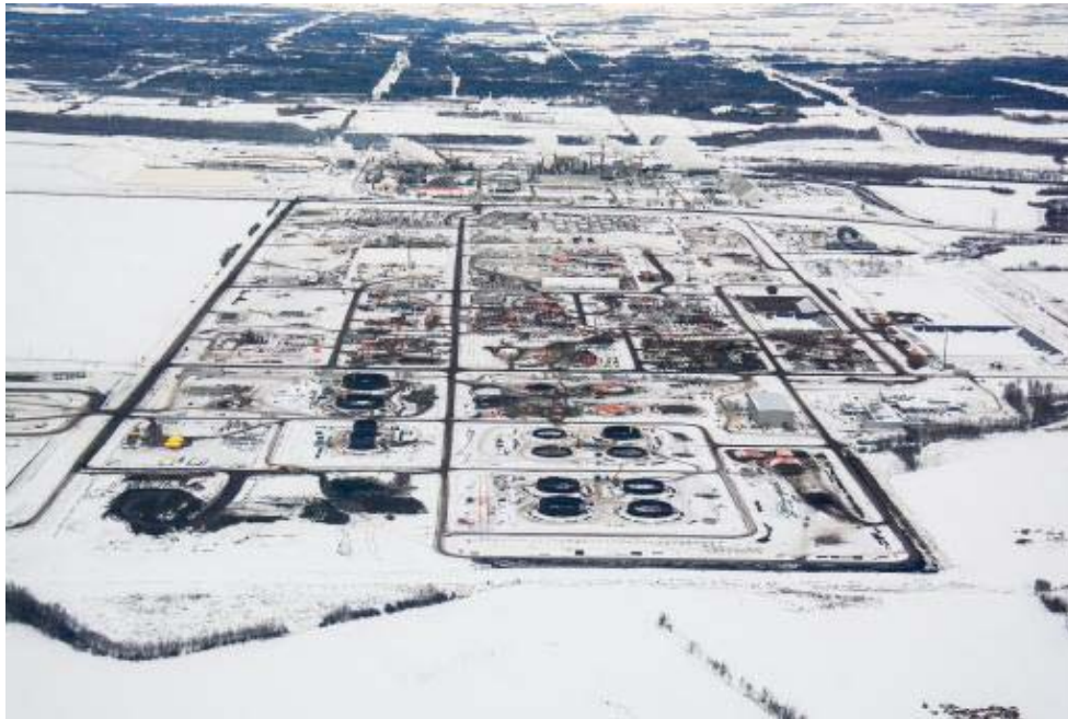
North West Redwater Partnership Sturgeon Refinery – Under construction
