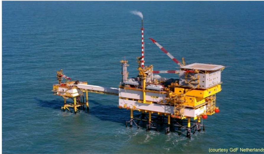
Figure 2. The K12-B offshore platform in the North Sea where CO 2 is injected into a sandstone formation containing natural gas. Source: co2geonet.com
