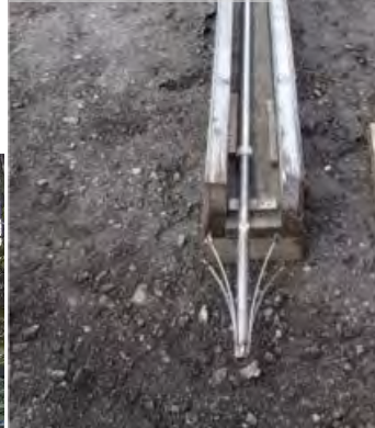
Terminal diffuser
