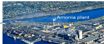
Yara Ammonia Plant - Porsgrunn
