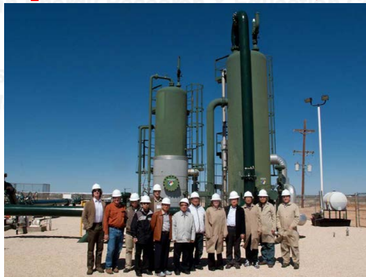
CO 2 separation unit for Tinsley
