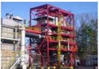
Alstom BSF Windsor US - 15 MWth Oxy - Coals
