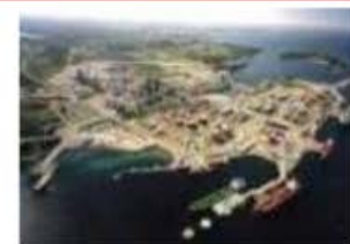
TCM Mongstad Norway - 40 MWth Chilled Ammonia - Gas
