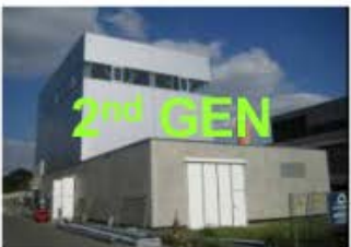
RFCS EU - Darmstadt Germany - 1 MWth Chemical looping - Coal
