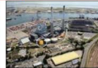
EDF - Le Havre France - 5 MWth Adv. Amines - Coal
