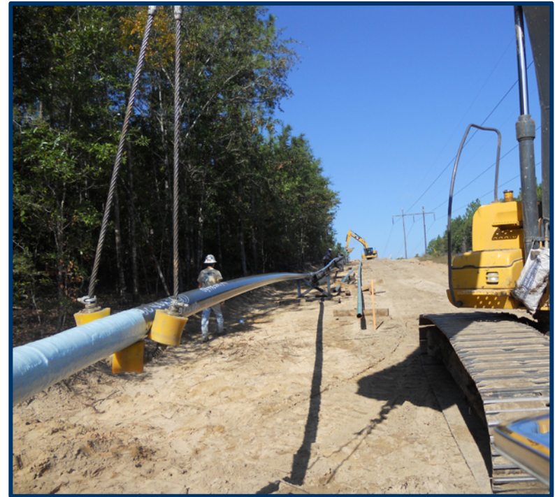
Handling pipe for horizontal directional drill
