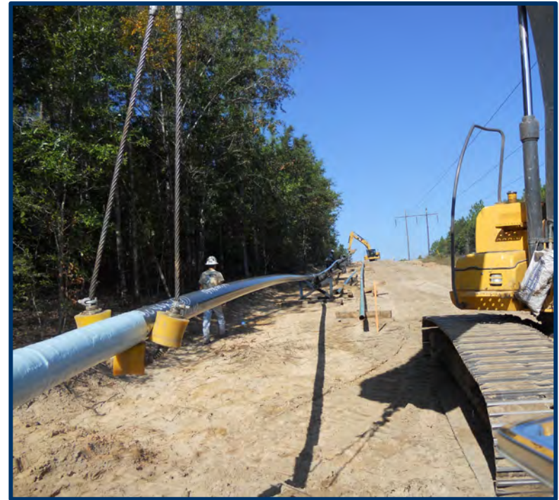
Handling pipe for horizontal directional drill
