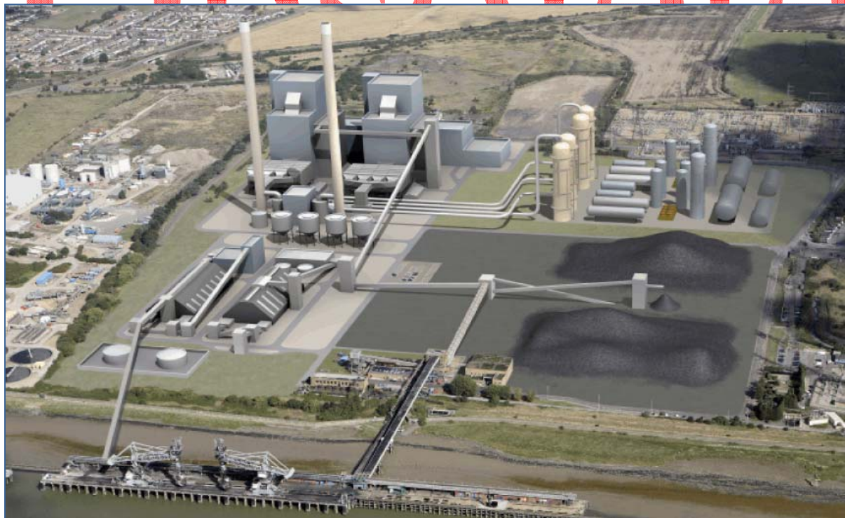
Figure 3. Photo montage of a 2x800 MW UK coal-fired power station with capture — shown behind the coal stockpiles (sourced from Imperial College, London and RWE Group)
