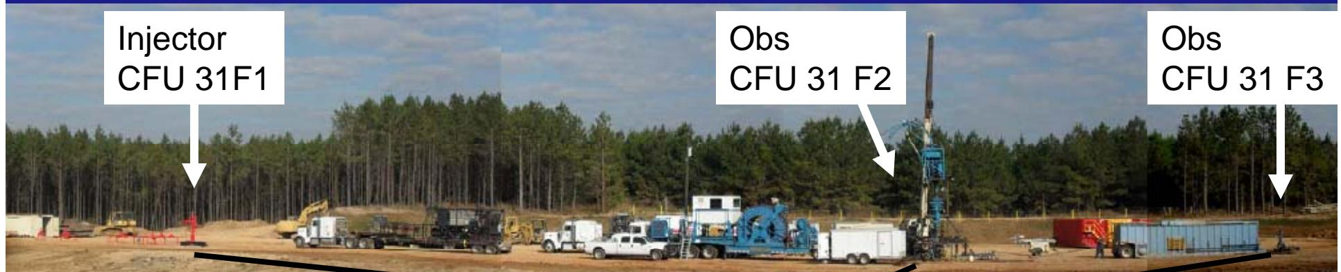
Closely spaced well array to examine flow in complex reservoir
