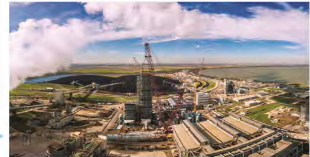
Sixteen-foot diameter ductwork takes flue gas from the coal plant to the carbon capture facility where the CO2 is removed from the flue gas by the amine solution in the tall absorption tower and then separated from the amine as 99.9% pure CO2 in the smaller regenerator tower to the right before being compressed and delivered to the oil field. (Photo: Business Wire)
