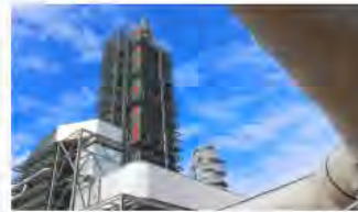
Sixteen-foot diameter ductwork takes flue gas from the coal plant to the carbon capture facility where the CO2 is removed from the flue gas by the amine solution in the tall absorption tower and then separated from the amine as 99.9% pure CO2 in the smaller regenerator tower to the right before being compressed and delivered to the oil field. (Photo: Business Wire)
