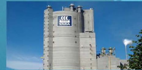
Yara Porsgrunn Ammonia production
