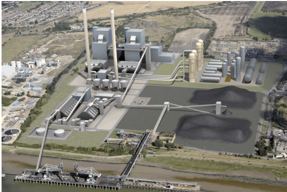
Figure 3. Photo montage of a 2x800 MW UK coal-fired power station with capture – shown behind the coal stockpiles (sourced from Imperial College, London and RWE Group)
