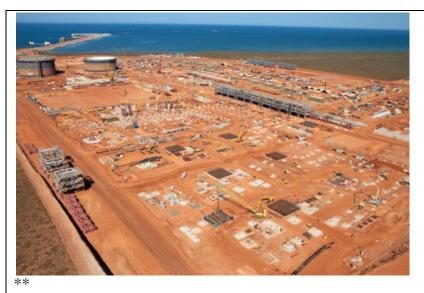
The Marine Offloading Facility (MOF) extending from the gas plant footprint. The MOF will enable the offloading of materials required for the Gorgon Project.
