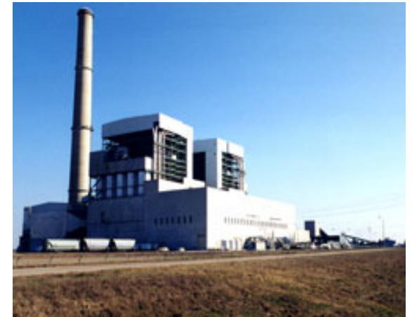
Northeastern Plant - Oologah, OK
