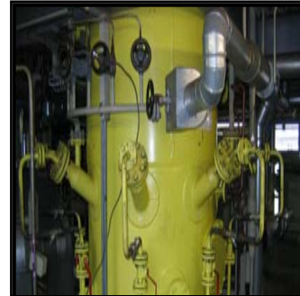
Gasified in Freiberg
