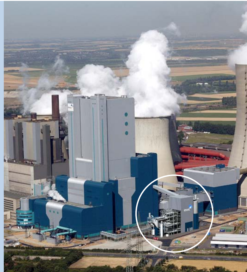
Prototype WTA coal-drying plant at Niederaußem BoA
