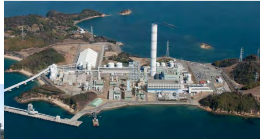
Osaki CoolGen (OCG) IGCC Demonstration Plant (1,180t/d / 2016~ / Osaki)
