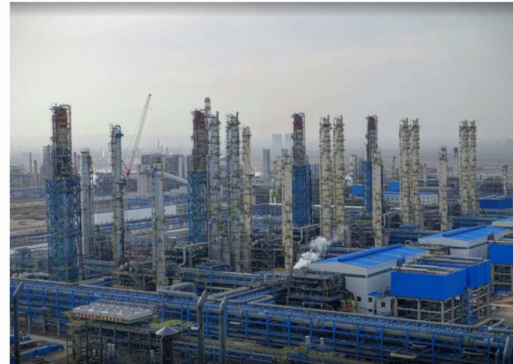
Shenhua Rectisol Plant in Ningxia, China Four Trains: 1.12MM Nm 3 /h each Startup: June 2016
