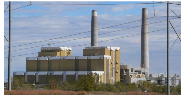
Gerald Gentleman Station (NE)
