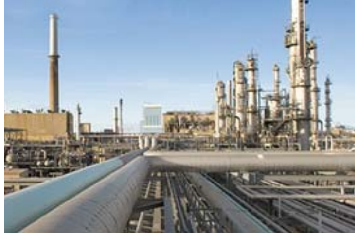
Dakota Gas captures and sells CO 2 produced at the Great Plains Synfuels Plant to two customers and transports it through a 205-mile pipeline to Saskatchewan, Canada, to be used for enhanced oil recovery (EOR) in the Weyburn and Midale fields.
