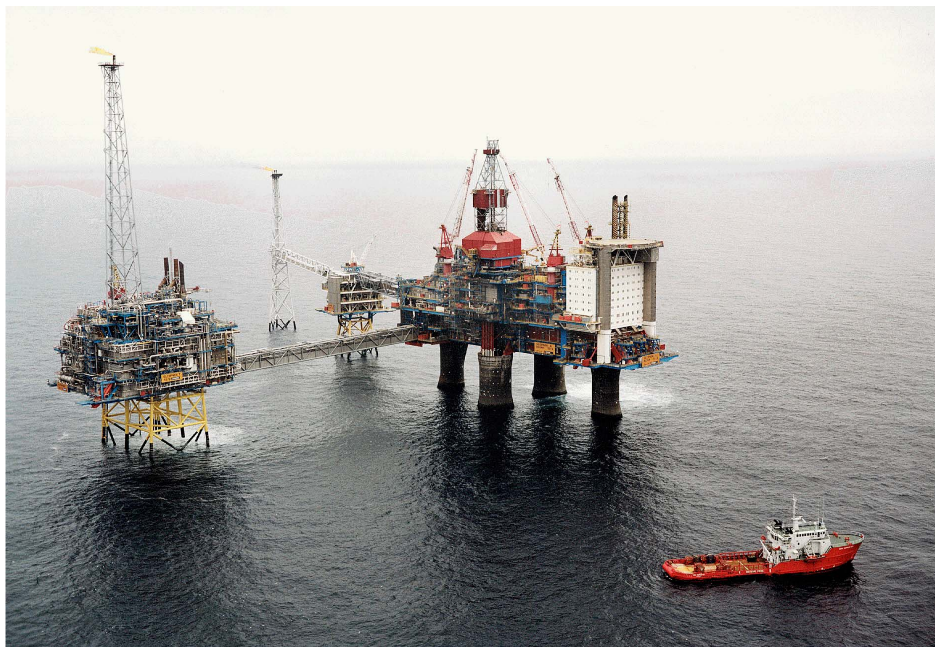
The Sleipner field – CO 2 Treatment and Injection. CO2STORE is a follow up and extension of the SACS Project (1998 – 2002)
