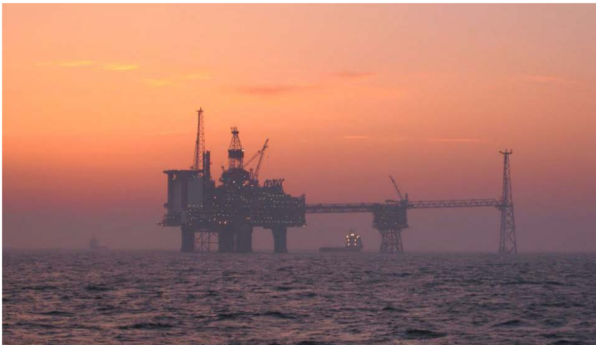
Figure 2-1: Sleipner CCS Facility (photo: Eiken, Statoil)
