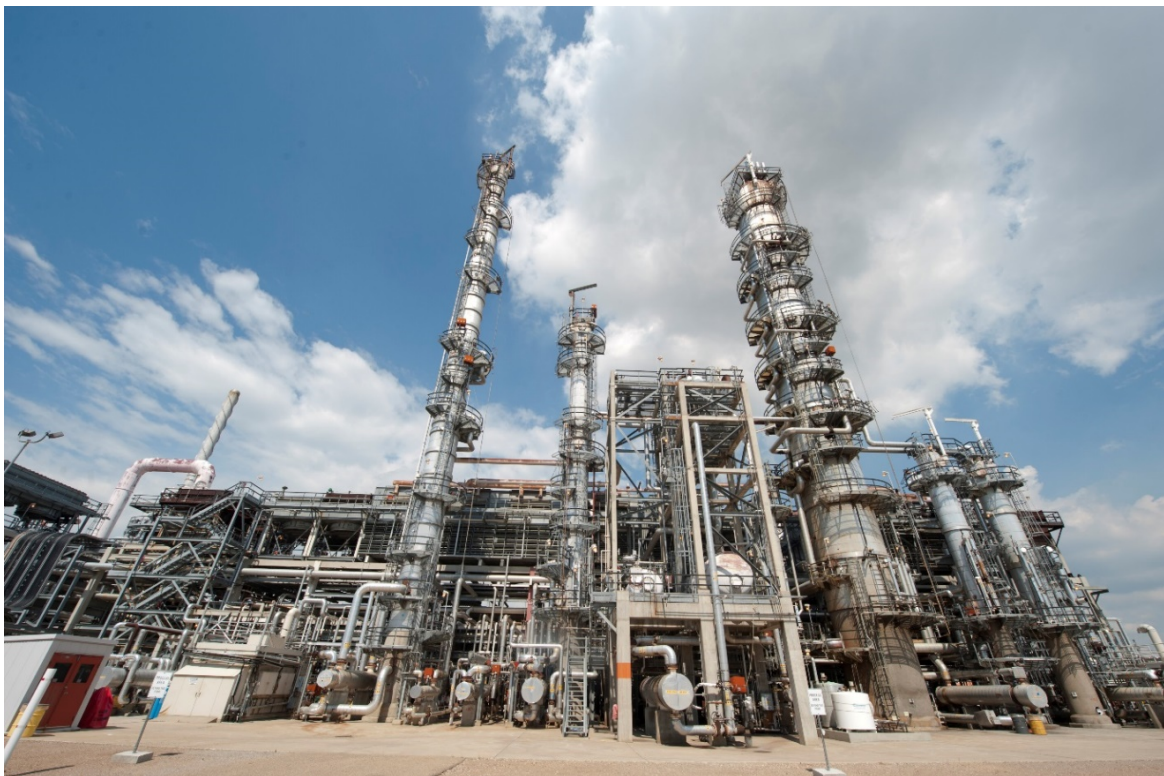
Figure 2-6: Quest CCS Facility at the Scotford Upgrader
