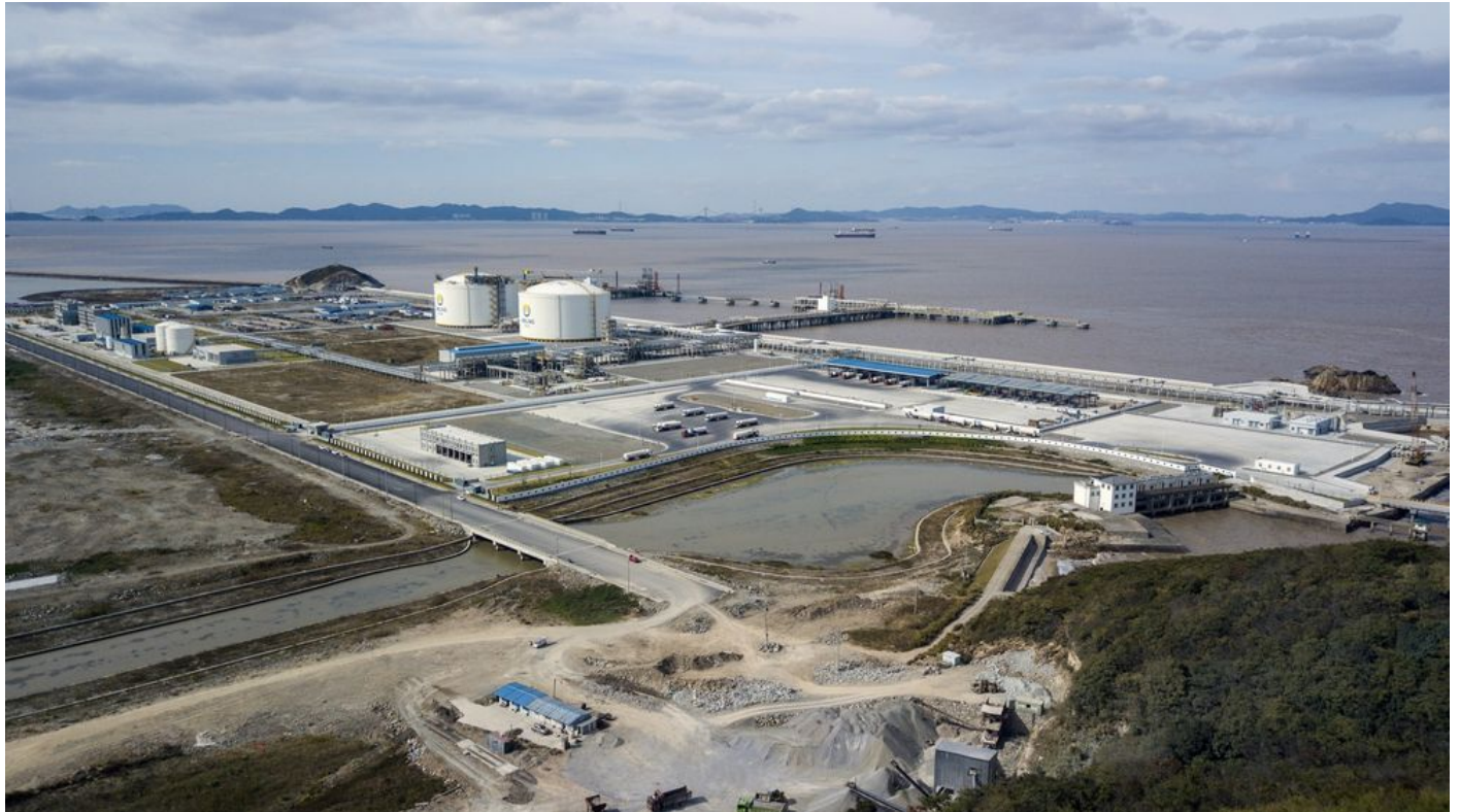
ENN Energy Holdings Ltd.'s LNG terminal on Zhoushan Island. Photographer: Qilai Shen/Bloomberg
