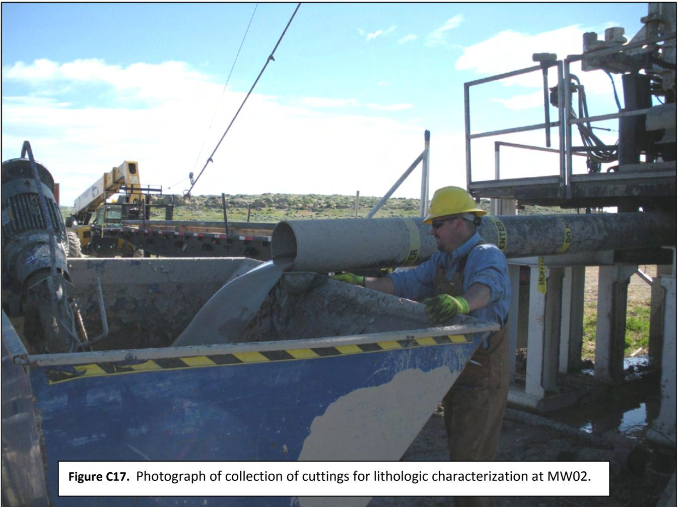
**Figure C17.** Photograph of collection of cuttings for lithologic characterization at MW02.
