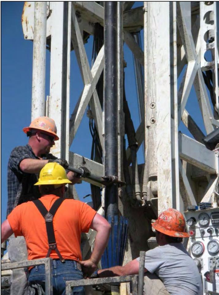
**Figure C21.** Photograph of securing sand basket and casing above screen.
