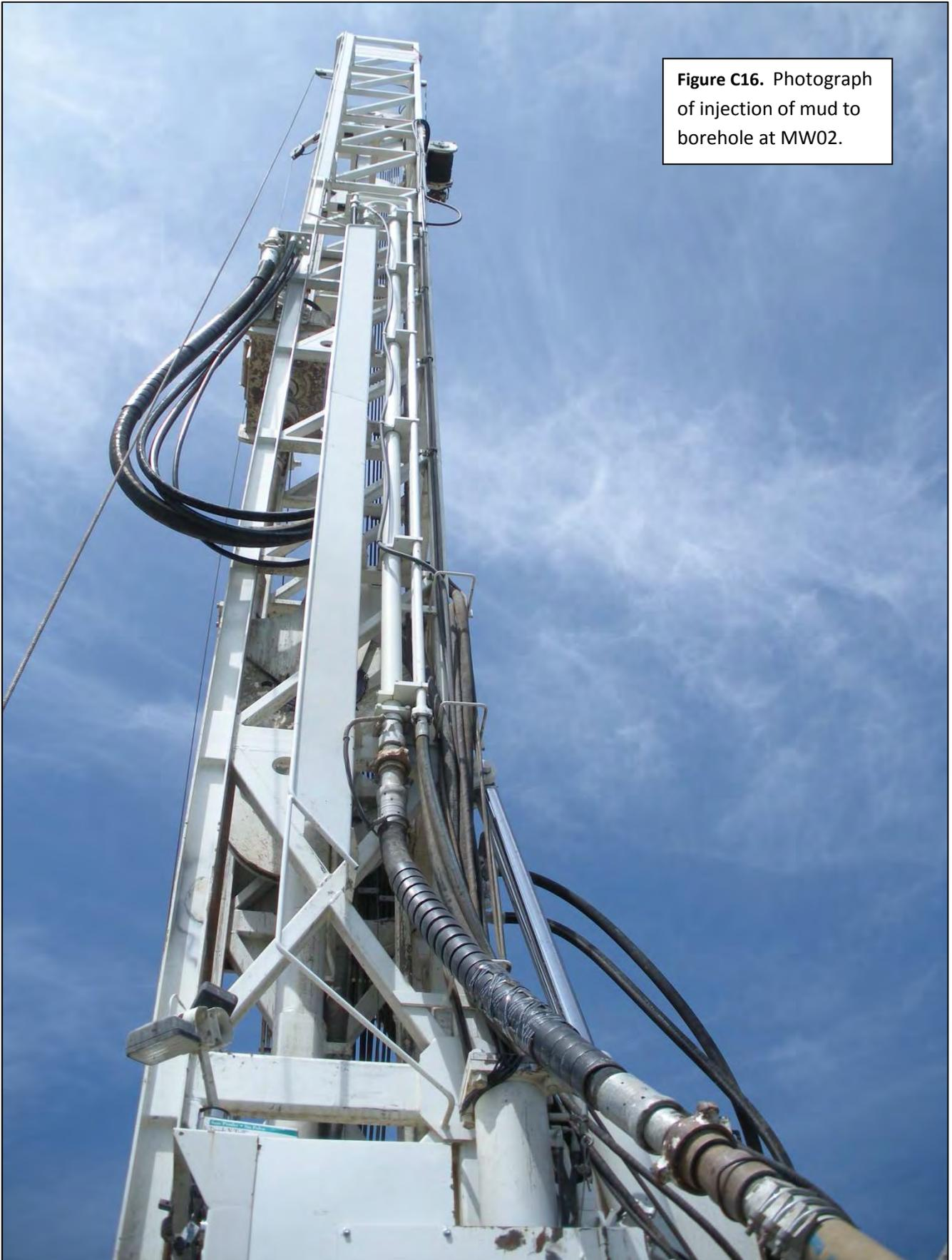
**Figure C16.** Photograph of injection of mud to borehole at MW02.
