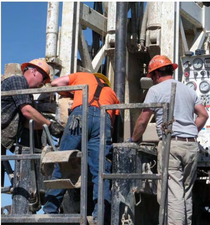
**Figure C22.** Photograph of placement of sand in sandbasket.
