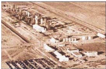
Brownsville, TX 7,000 bpd GTL Plant
