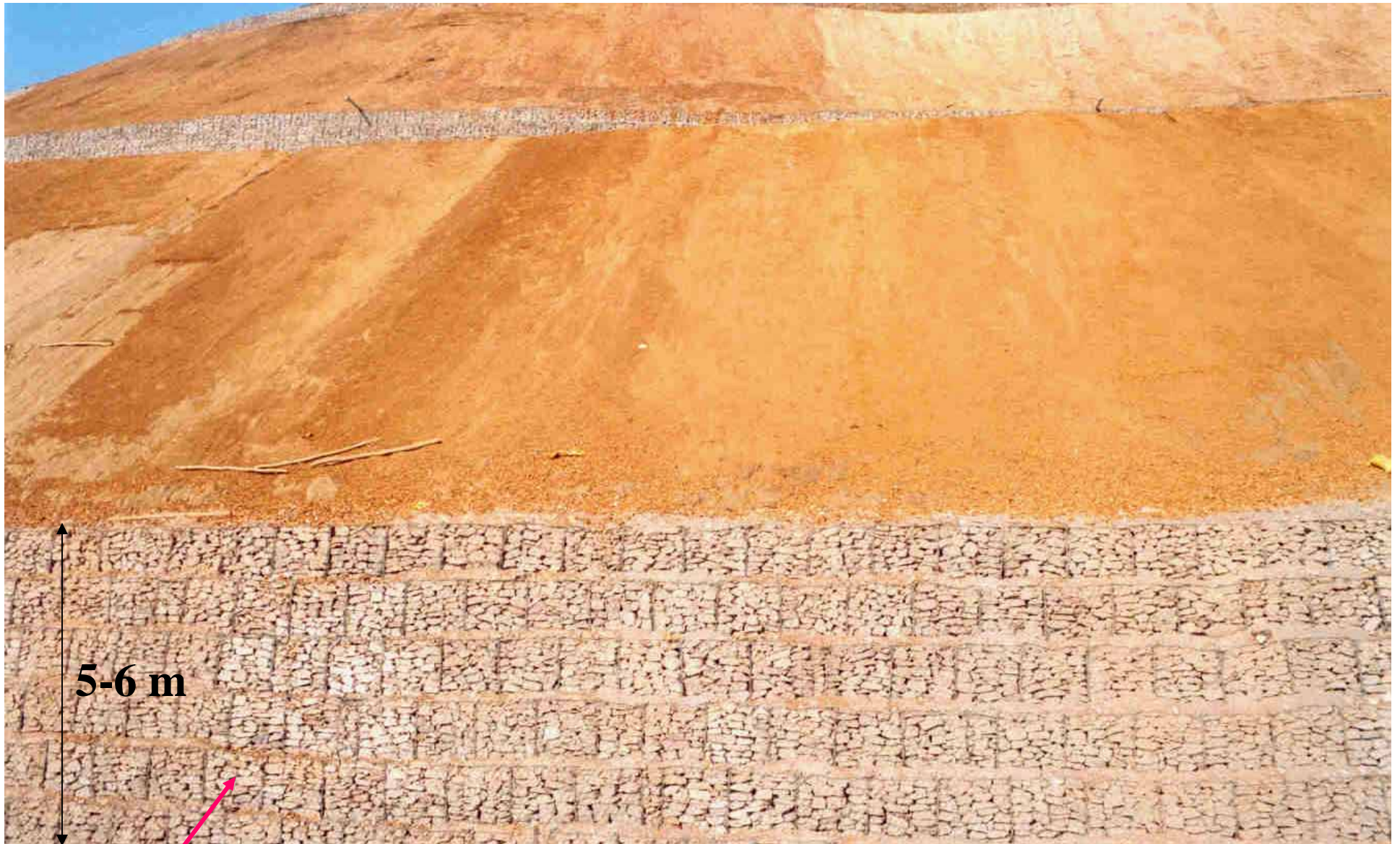
GABION WALLS AT THE TOE OF THE DUMP FOR ARRESTING THE SILT
