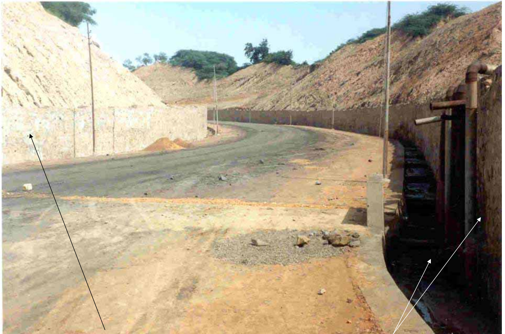
WALLS & DRAIN AT THE TOE OF THE DUMP FOR ARRESTING THE SILT
